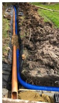
Ironically, a long conversation was had prior to work commencing about how best we could manage the drainage issues. Whilst not the cheapest option, we decided to install a substantial new drain at the top of the site. We could not have made a better decision as it turned out!
